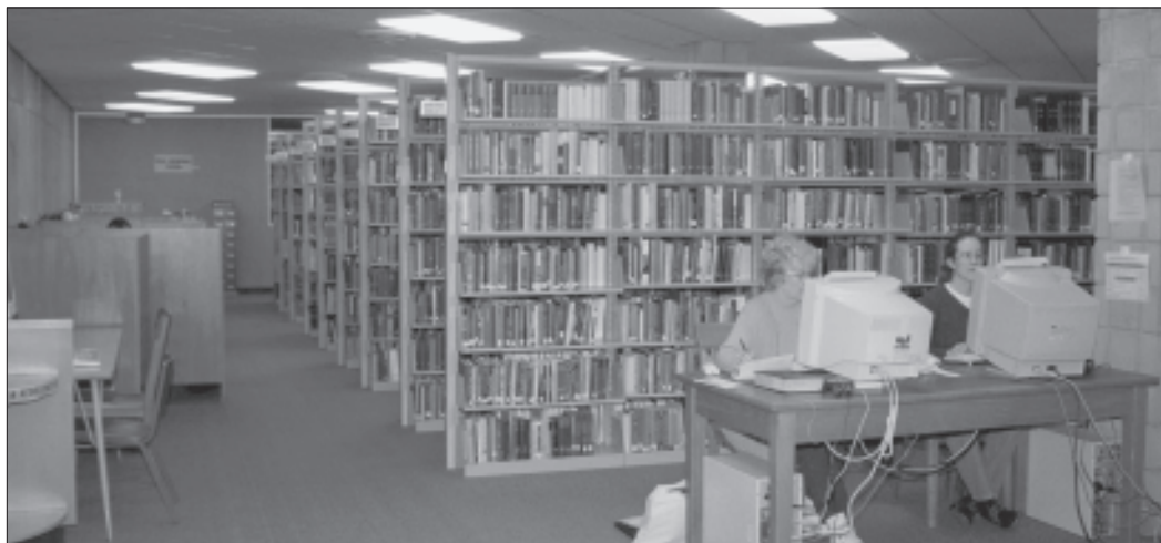
The AMBS library currently consists of a reading room and workroom that were part of the original 1958 structure, a basement area for periodical stacks and a separate underground room for book stacks. Limited space, water leakage during heavy rains and lack of comfortable work stations are some of the problems in the current bookstack area that make a new library facility a priority for AMBS.
