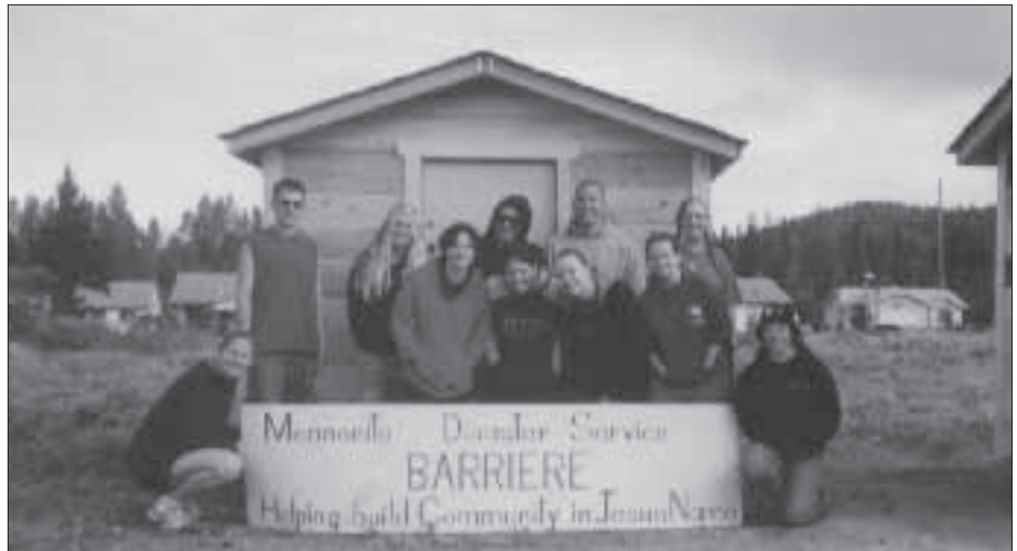
The youth of Coaldale Mennonite Church in Alberta recently spent a week in Barriere, B.C. doing forest fire cleanup and constructing four storage sheds. The highlight of the week was Friday evening, when some 60 residents gathered to express their gratitude to the group. Among the testimonies was an expression of regret from the man responsible for the fire. He thought he had put out his cigarette but he soon realized he had started a fire that could not be contained. As a result of this tragedy he became a Christian. The youth, from left: Bonnie Dyck, Nathaniel Nickel, Megan Dyck, Lynette Wall, Joel Penner, Bonnie Quinn, Tessa Janzen, Mark Dyck (group leader), Jennifer Giesbrecht, Christina Nickel, Vickie Giesbrecht. Earlier in the year John and Alice Klassen contributed 10 days of voluntary service at Barriere as well.—Olga Epp
