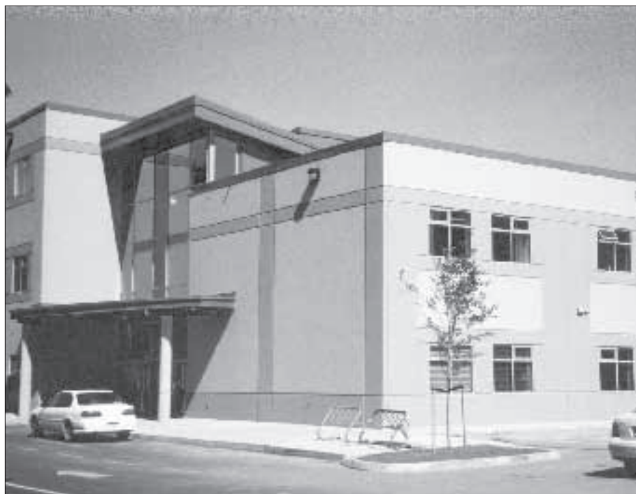
The new middle school at MEI received students this fall.
