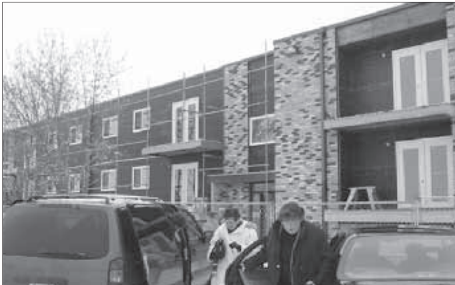
The first apartment block is almost ready for “re-peopling.”
