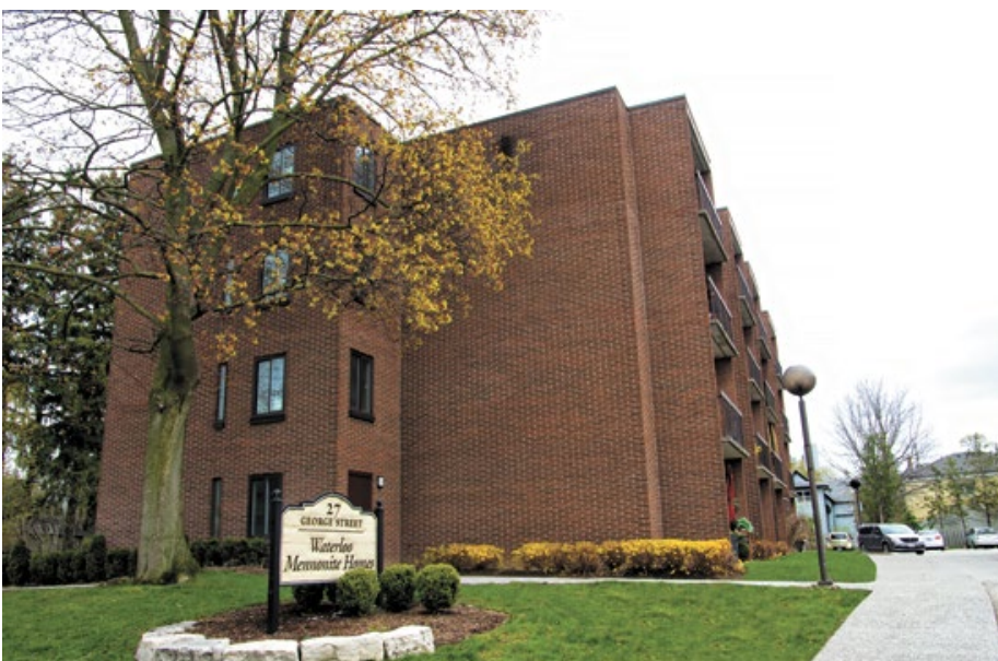
WATERLOO MENNONITE HOMES PHOTO
