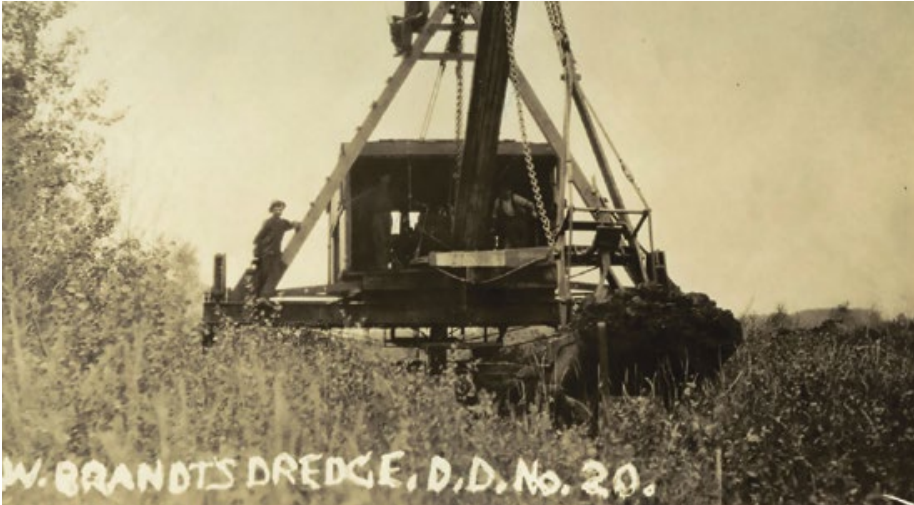
Klaas W. Brandt's dredge used to construct the aqueduct.
