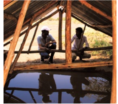
Sisay Kasu, left, project manager for MCC Ethiopia, and Hussien Edris, project co-ordinator for Afar Pastoralist Development Association (APDA), look at the sediment trap leading into a birkat, a traditional water catchment system that MCC and APDA have expanded and modernized as part of an emergency water project in northern Ethiopia.
