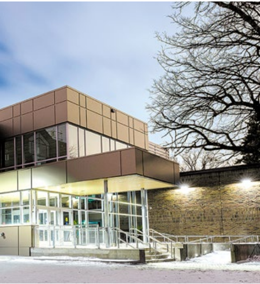
PHOTOS COURTESY OF WESTGATE MENNONITE COLLEGIATE ate, features an atrium at the front.
