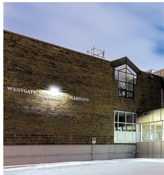
PHOTO BY NICOLIEN KLASSEN-WIEBE The newly renovated Westgate Mennonite Collegiate
