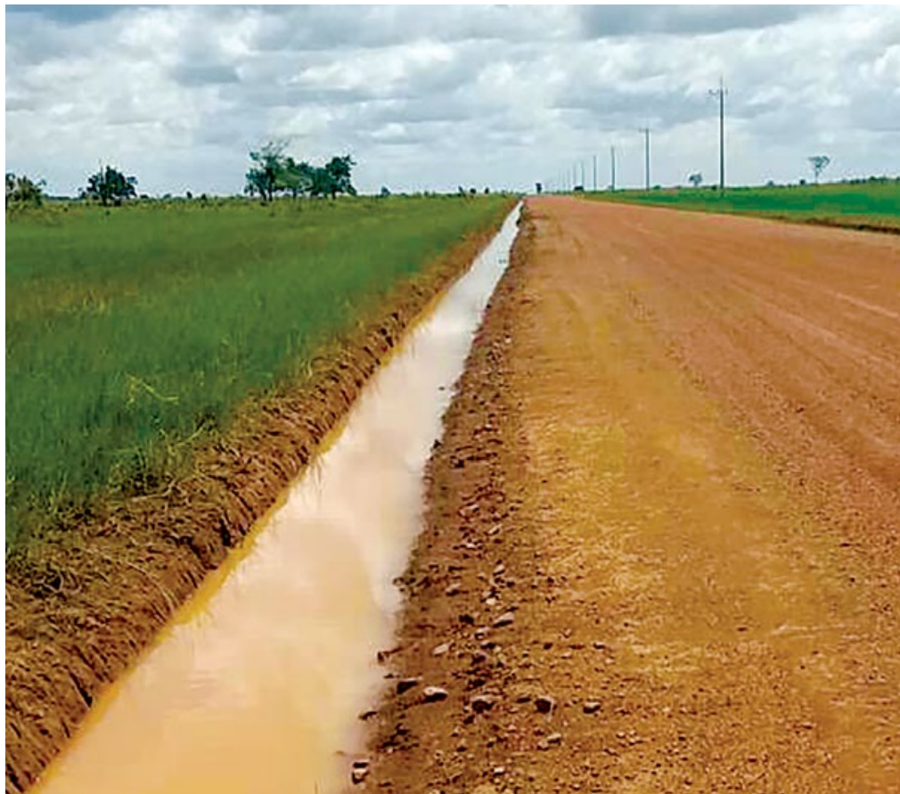
A new road and hydro line in the Liviney Colony.
