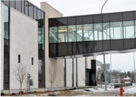
A new pedestrian bridge links CMU's north and south campuses.
