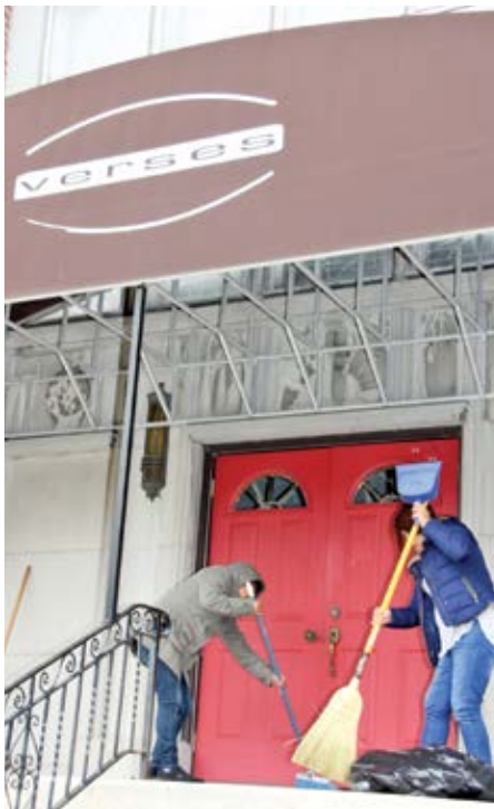
While it still said Verses Restaurant on Oct. 25, the building is being cleaned and prepared to be the Chin Christian Church place of worship and work.
