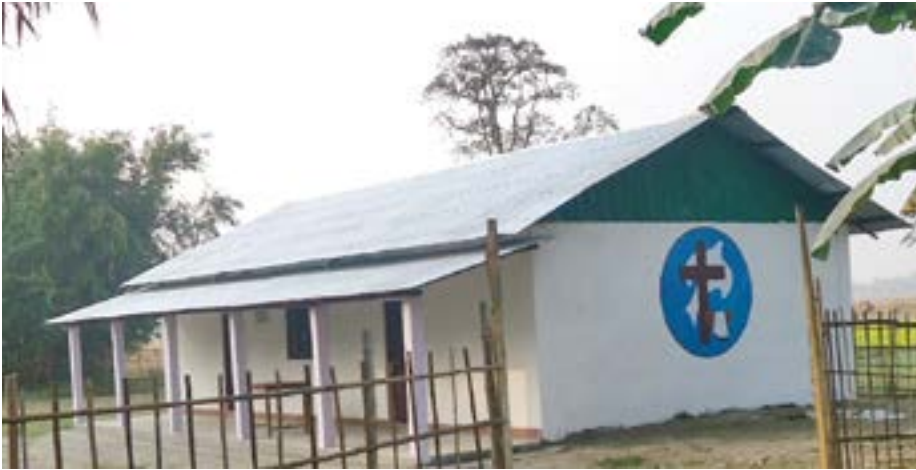
A concrete building was constructed by Behelwa Brethren in Christ (BIC) Church, Babiya, Nepal, with financial assistance from the Mennonite World Conference Global Church Sharing Fund.
