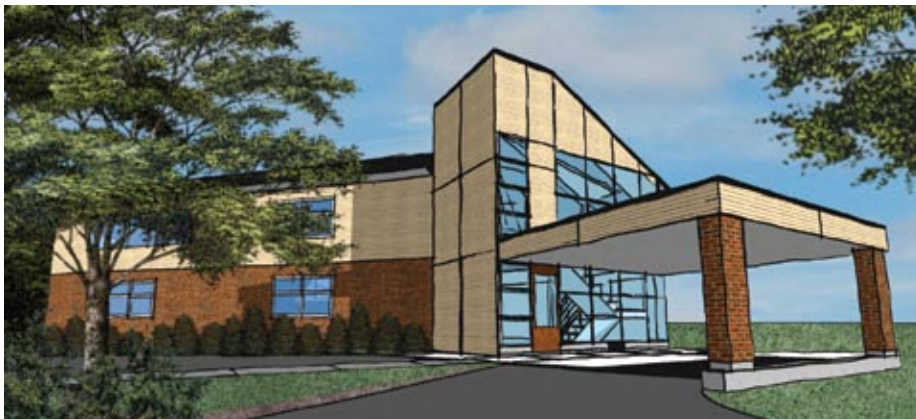
The new "Under One Roof" House of Friendship facility for addictions is a building to be renovated at 71 Ann Street, Kitchener, where the footprint of the building will be maintained, while the existing second floor will be extended across the entire building, adding 2,500 sq. ft., to the current 12,000 sq. ft.—a $2 million project.
