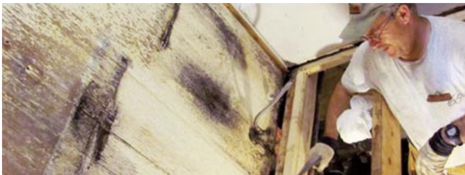
Mark Bauman of St. Jacobs Mennonite Church, Ont., removes mouldy wood and materials before rebuilding a floor in an Attawapiskat First Nation home this spring.
