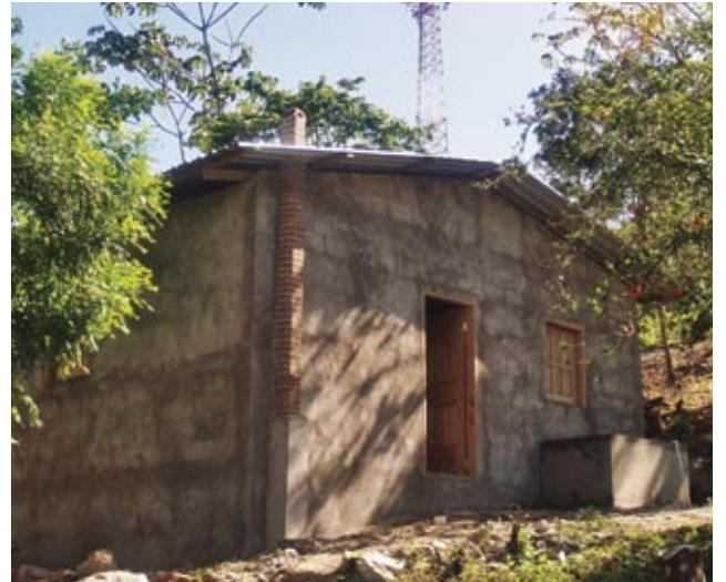
The villagers' new homes are two-bedroom, concrete-block structures, complete with indoor plumbing and running water, a kitchen and family room. The villagers made the blocks themselves, working from a mould they purchased.
