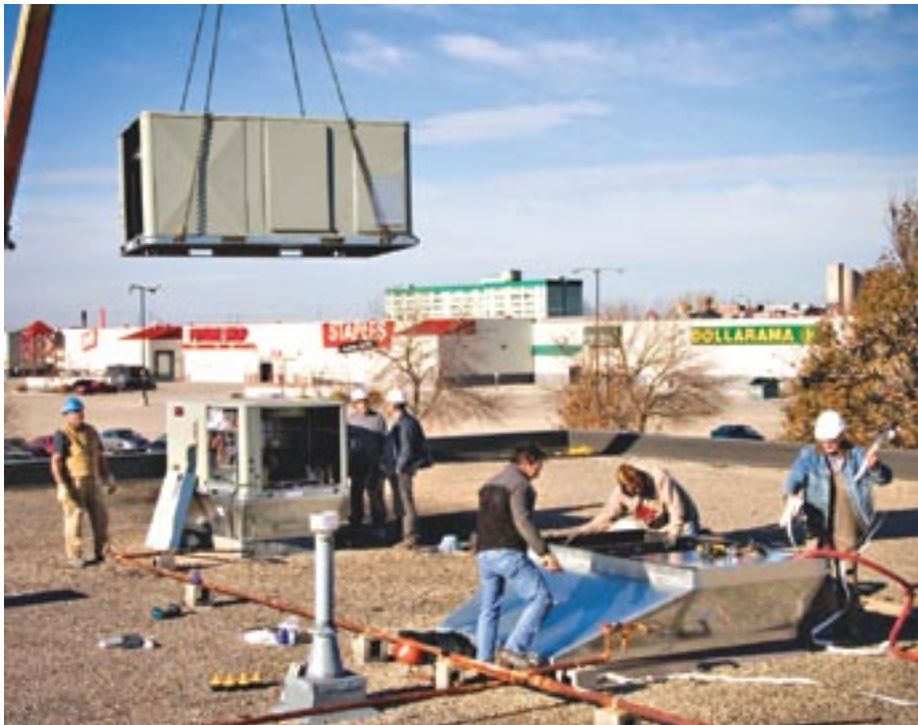
Mennonite Central Committee Canada’s Winnipeg headquarters had geothermal heating installed in October 2008 in order to reduce the carbon emissions it takes to heat the office building.
