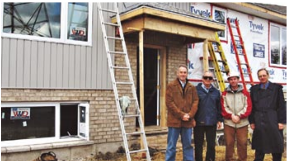
Peter Janzen and Bill Devolin from Niagara United Menonite Church, Niagara-on-the-Lake, Ont., are pictured with Alastair Davis, Habitat Niagara CEO, and John Sherk, construction teacher with the District School Board of Niagara, at the site of a Habitat for Humanity building project in St. Catharines the church financially supported through its missions committee. The house was completed in February.
