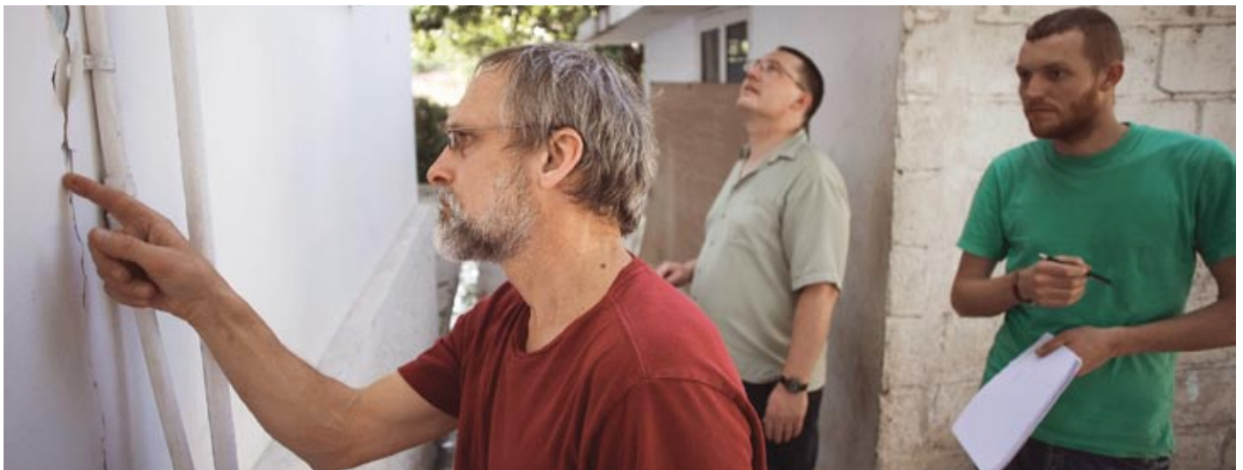
From left to right, volunteer engineers Johann Zimmermann, Peter Pereverzoff and Marcus Schiere begin their work in Haiti by inspecting the structural integrity of the Mennonite Central Committee offices in Port-au-Prince, where a 7.0 magnitude earthquake damaged much of the capital city on Jan. 12.
