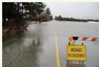
A flooded road in Chilliwack.
