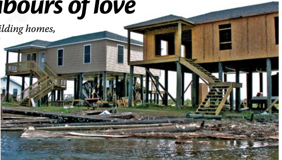
Mennonite Disaster Service houses stand four metres above the ground at water’s edge at Grand Bayou, La., a fishing village about 35 miles south of New Orleans.
