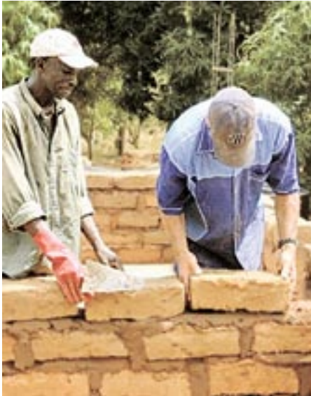
Yacouba, the head mason, left, teaches Norm Nicolson how to lay bricks.
