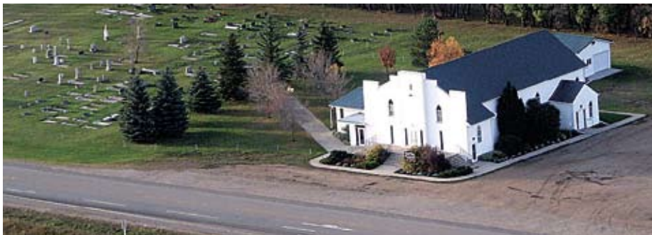
Eigenheim Mennonite Church as it currently stands is to be rebuilt in another location to alleviate a number of problems, including flooding and problems some congregants have using the chair lift that leads to the basement. The new church will be built on one level.
