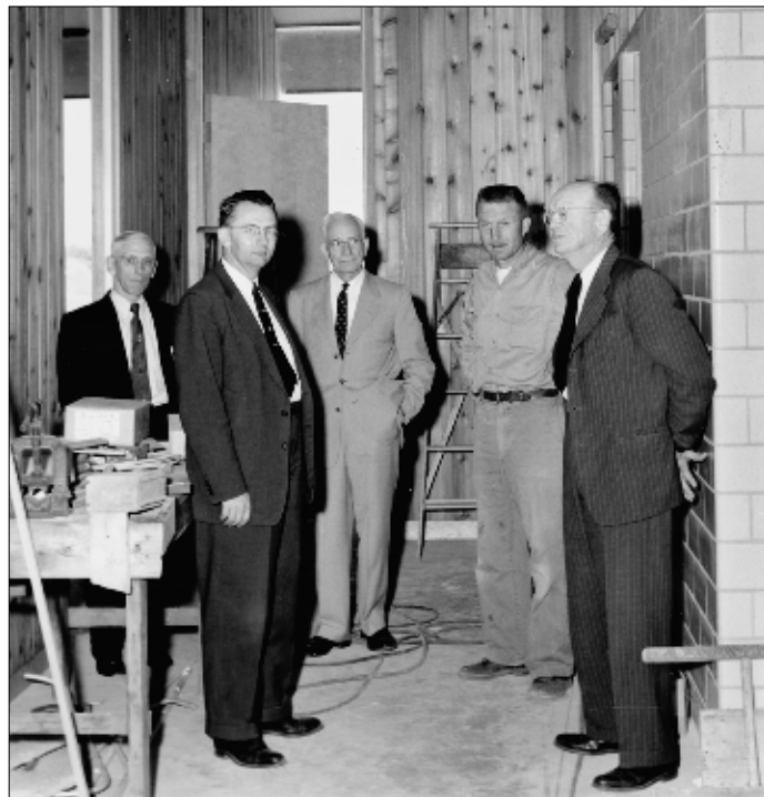
The executive committee of the MBS board checks on the progress of construction on the Elkhart campus, May 28, 1958: R.L. Hartzler, Erland Waltner, J.N. Smucker, Henry Knuck (contractor), A.E. Kreider.
