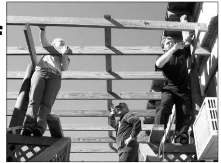
Members of Herschel Ebenfeld Church helped rebuild New Beginnings Church.
