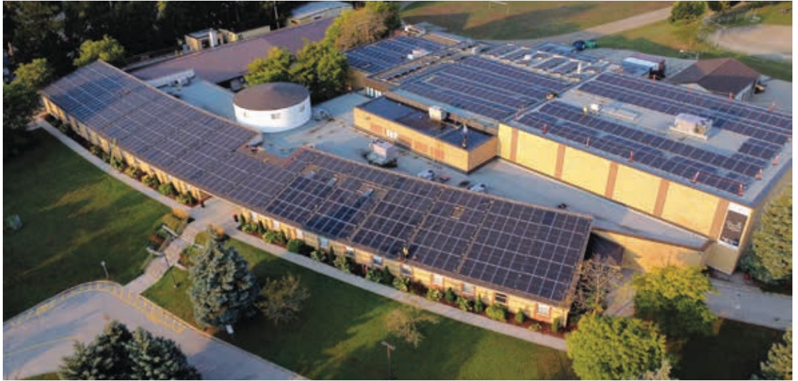
Aerial image of Rockway’s roof covered with 875 solar panels.
