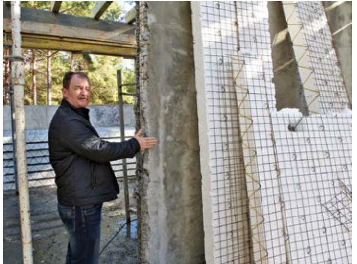
*As a bi-vocational pastor, Sergey Deynekin makes styrofoam and wire building panels in his backyard. Once the panels are erected, they are covered with concrete stucco. The resulting structure is sturdy and cost-effective. Deynekin plans to use his panels to build a new home for Chernobaevka Church.*
